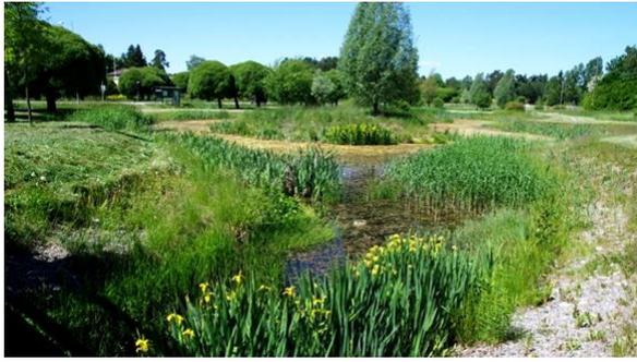
In ponds, pollutant removal is mainly achieved by the sedimentation of particle-bound compounds. Further removal can be achieved by increasing the biomass in and around the pond, as the vegetation and biological processes can reduce the concentrations of dissolved pollutants. Therefore, wetlands
