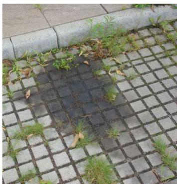
As an alternative to traditional asphalt and concrete surfaces, different kinds of permeable surfaces can be used which still have enough bearing capacity for vehicles but at the same time allow water to infiltrate instead of running off. Gravel, permeable pavers, permeable asphalt and paving with permeable joints are some examples.
