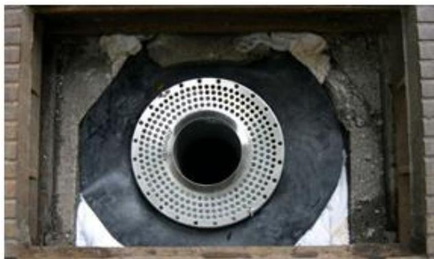
Filters can be installed in existing stormwater drains and can therefore be an option in already densely urbanized areas. They are most applicable in areas with moderate to high contaminant loads and places that lack the spatial requirements for the implementation of other techniques, such as for instance
