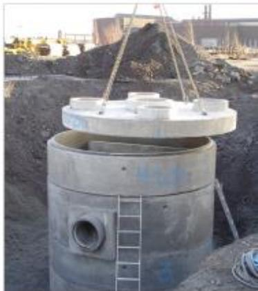
Oil separators are mainly designed to remove higher concentrations of oil contaminants and their removal efficiencies for lower concentrations of oil and other volatile pollutants are limited. They are suitable as a complement to other stormwater facilities where there is a need of protection against temporary, larger spills of oil; for instance, at bigger parking areas or fuel stations.
