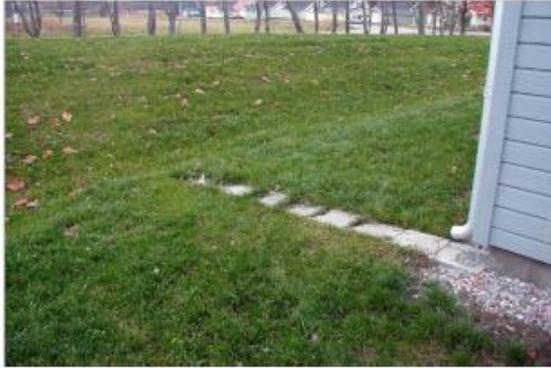
A simple, robust and cost-effective measure to detain and clean stormwater is to spread it out on a green surface. Here, both the vegetation and the soil contribute to flow reduction and pollutant removal of stormwater diverted from close-by roads, streets, parking lots, roofs and residential courtyards. It is desirable that the top soil layer has a high infiltration
