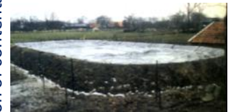
Covered lagoon for slurry.
