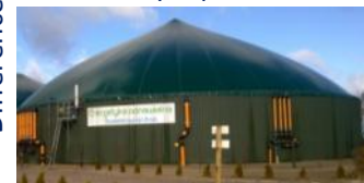
The biogas plant.
